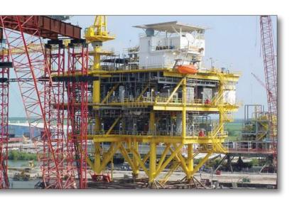
Dynamic was contracted by Enterprise to fabricate and hook-up the Ship Shoal 332 B platform and the High Island A5C platform for the CHOPS project. 3 topside components of 3,500 tons, 2,500 tons and 1,500 tons were fabricated and loaded out. To meet the aggressive schedule, Dynamic worked almost 600,000 man hours, a 24/7 effort, without incident and accident free.
