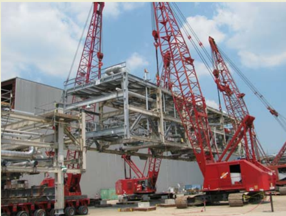
GOHT Modules being stacked for loadout
